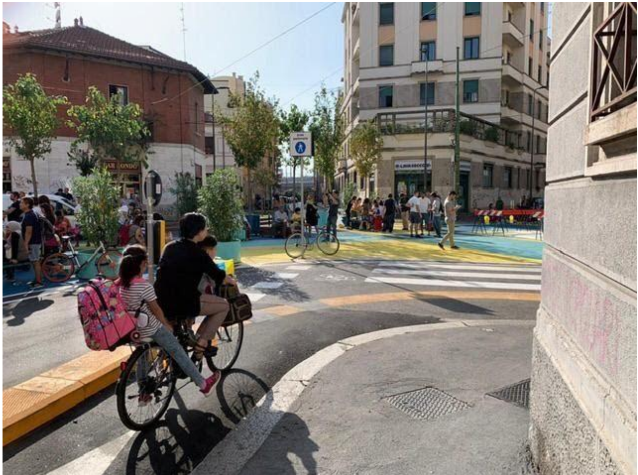
Milan: "Piazze Aperte". A cycle lane Contraflow, delimited by a bollard, in Via Martiri Oscuri.
