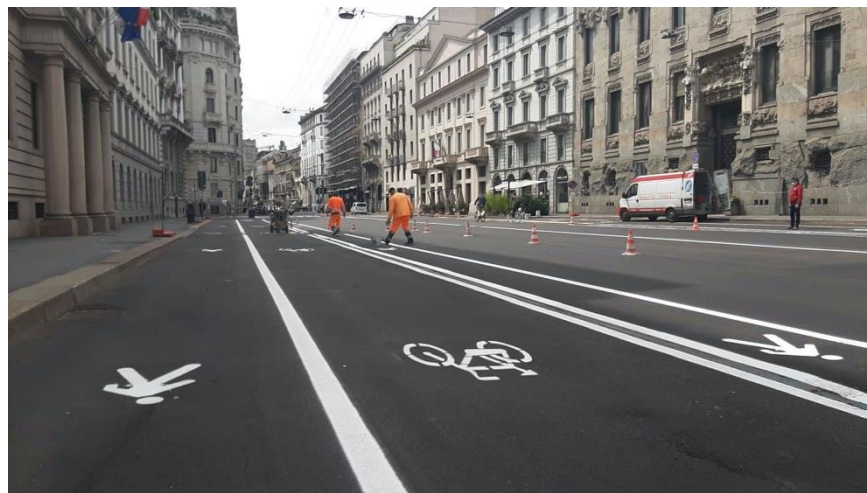
Construction works for the new cycle lane on Corso Venezia (04/30/2020)
